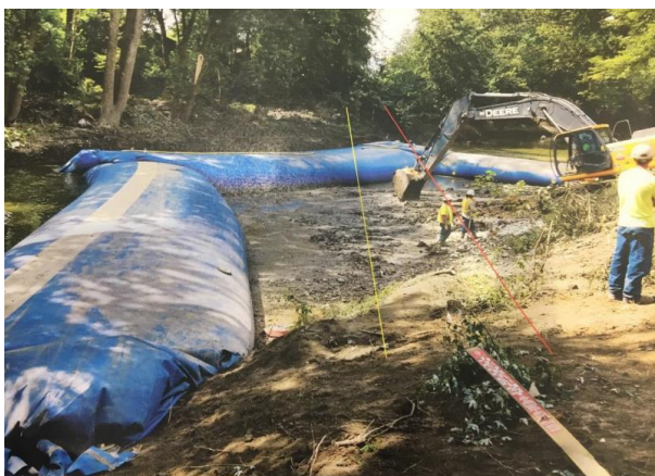
Figure 1 Bladder Dam Installation
