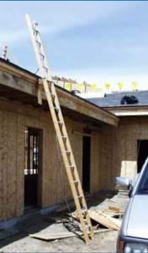
Proper ladder set-up
