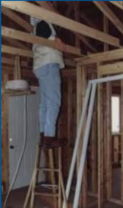
step ladder too short for this job
