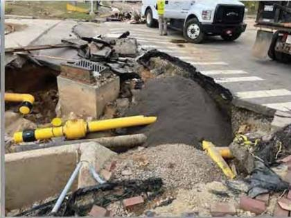
Rock Screenings were used to stabilize exposed pipe
